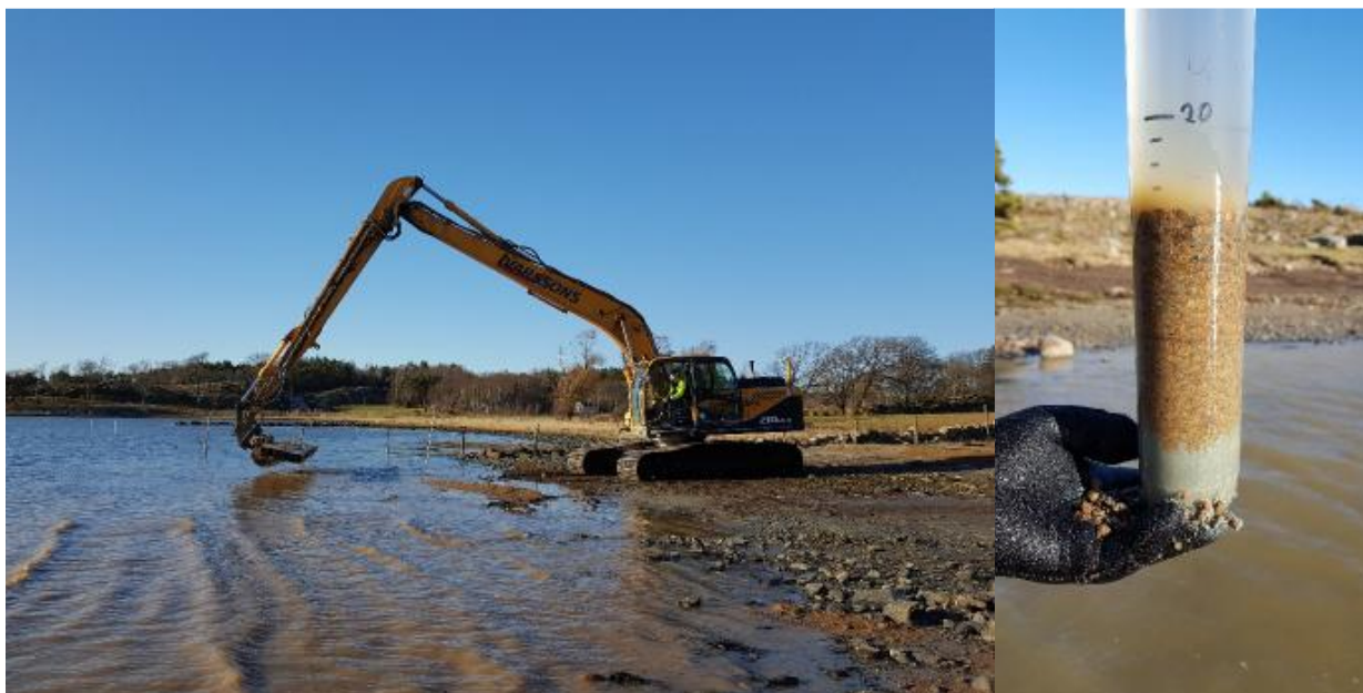
Figure 5.8. Sand capping at Lilla Askerön in March 2020 using an excavator from land. The right image shows a sediment sample from the sand-covered area, where the placed sand is clearly visible on top of the natural, muddy sediment.
