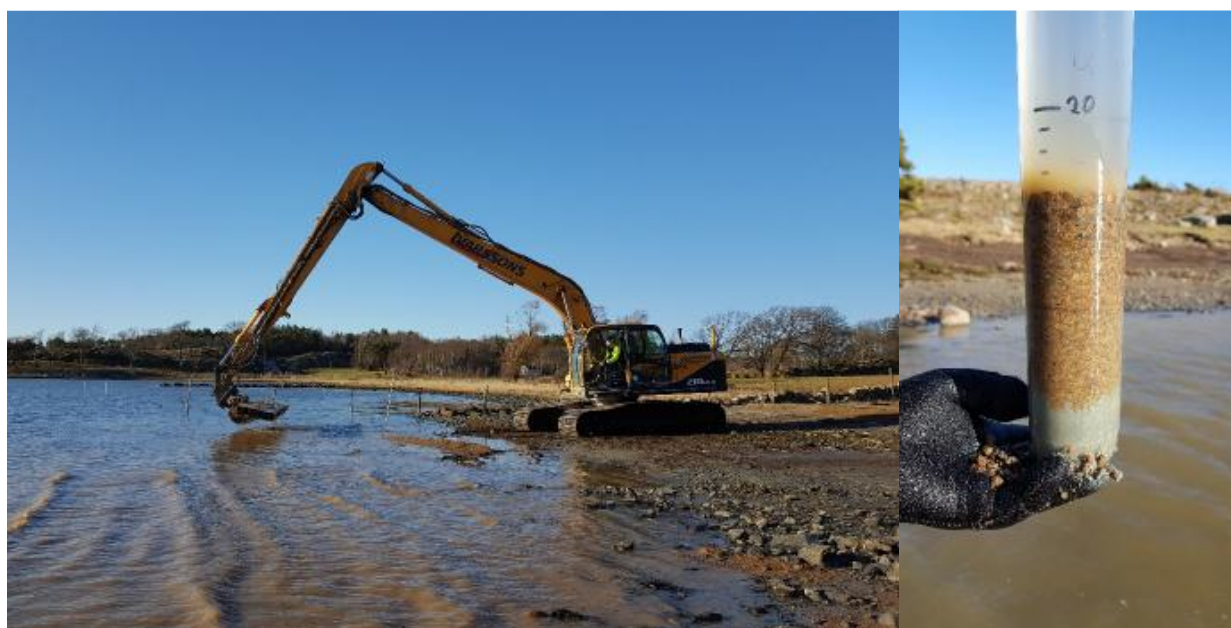
Figure 5.8. Sand capping at Lilla Askerön in March 2020 using an excavator from land. The right image shows a sediment sample from the sand-covered area, where the placed sand is clearly visible on top of the natural, muddy sediment.
