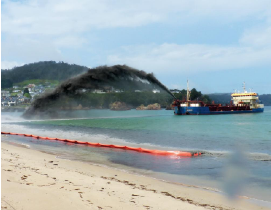
Figure 6. Beach nourishment using the rainbowing method, where sand mixed with water is sprayed from the dredger (Image from Rohde Nielsen 2020).
