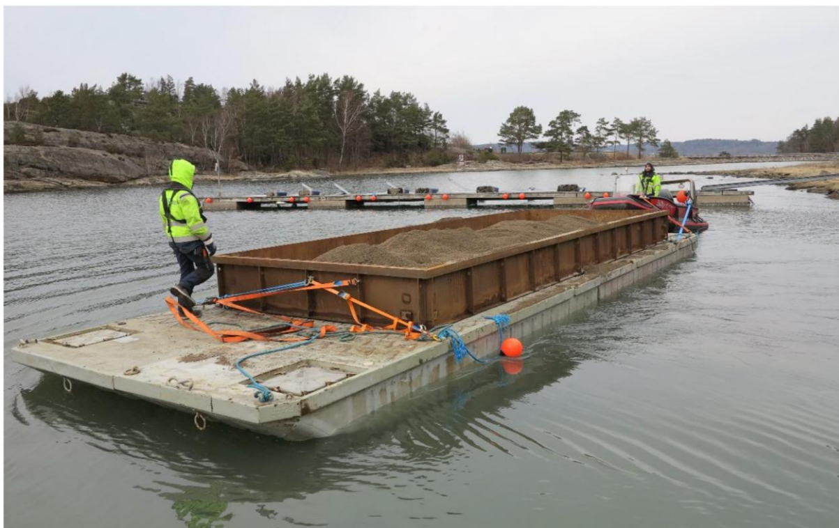
Figure 1. Transport of sand capping material on a barge towed by smaller workboats (Blue Orbis 2021).
