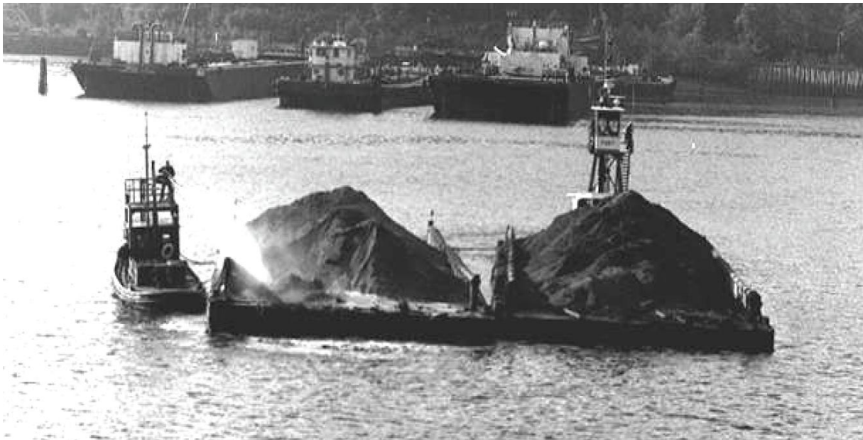
Figur 4. Hydraulic wasing of coarse sand into the water from sand piled on top of barges (figur från Bailey m.fl. 2005).
