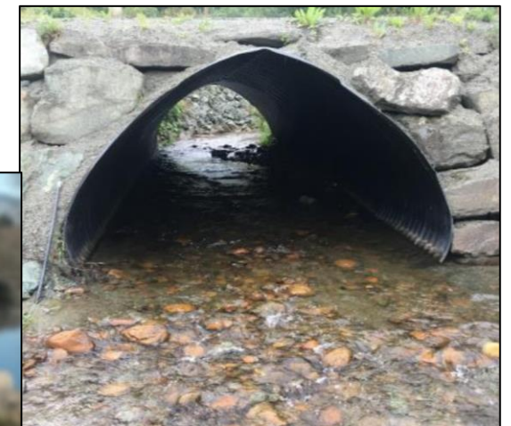
Culvert that allows fish/fauna passage. Photo: Morten André Bergan.
